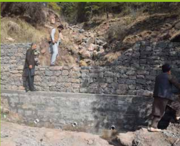
One of the dams we built in Azad Jammu and Kashmir to better protect homes and livelihoods.
